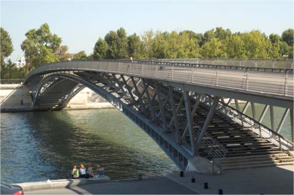
(Two bridges in one over the Seine – you can enter from the top level, or from the bottom and come up in the middle.)
